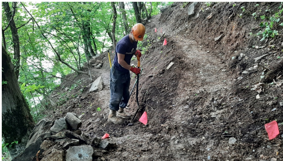
Constructing a new switchback in Lagodekhi National Park.
